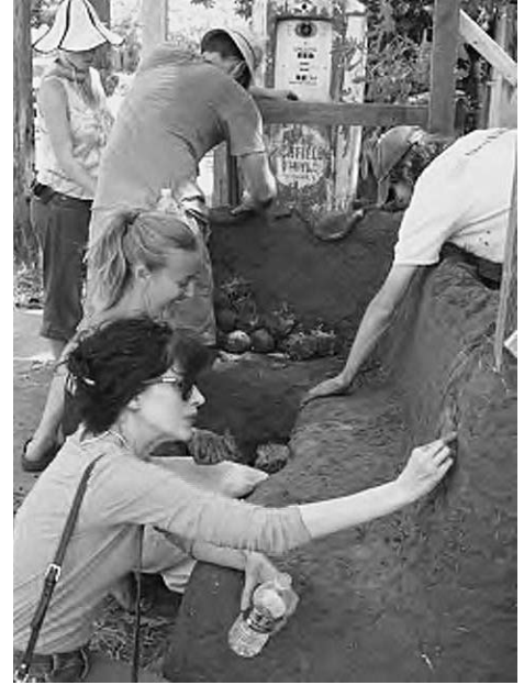
Building a cob bench at the new park on Joseph Street
